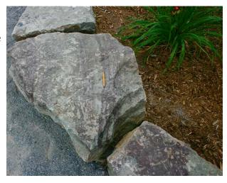
6 Most of these blocks of sandstone and limestone (see next page) that form the retaining wall behind the Crystal Palace display abundant stylolites. The tops of several capstones show many parallel striae, indicating that they came from a glacial pavement. The wall was built in the late 1800s when the area was heavily used for commercial purposes,
